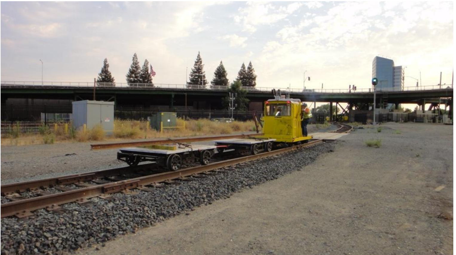
Finally, the UP Main has cleared. Mike H. and Frank in the Kalamazoo pull the new stick of rail over to Old Sacramento
