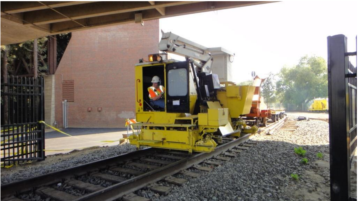
Heather pilots the man-lift over to the Shops pulling the chipper and flatcars with the extra rail
