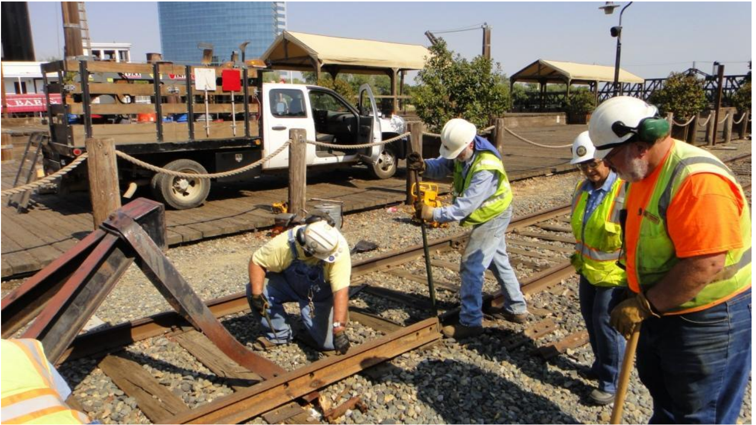
Mike F. and Mike M. shimmy the new rail into position
