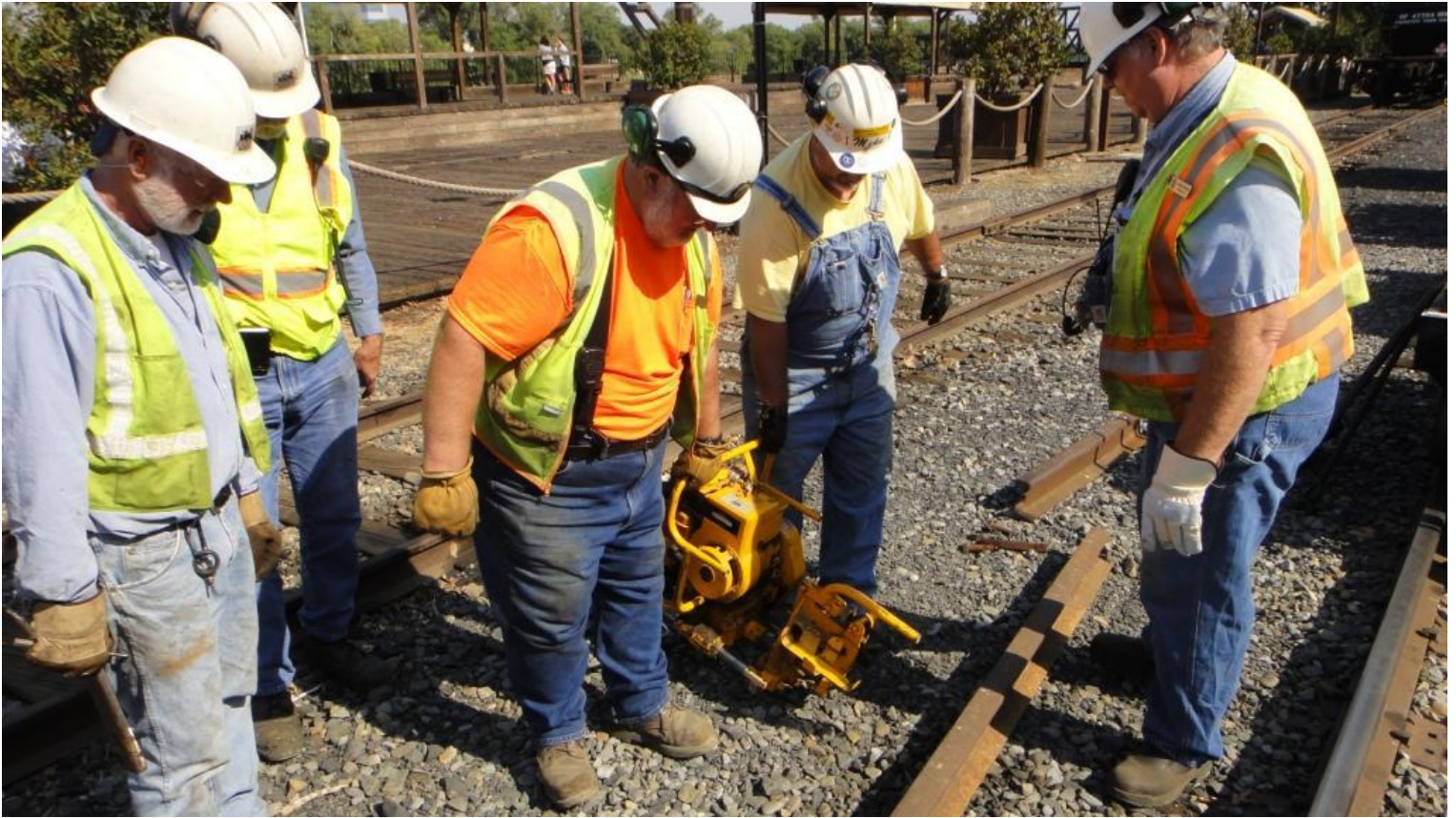
Frank and Mike F. bring in the rail-drill to make new bolt holes for the bumper's brackets
