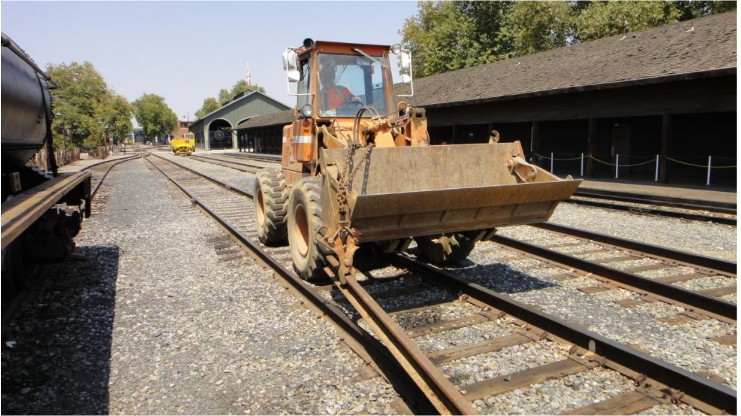
Frank drags the remaining rail to a position where it could be loaded onto a flat car
