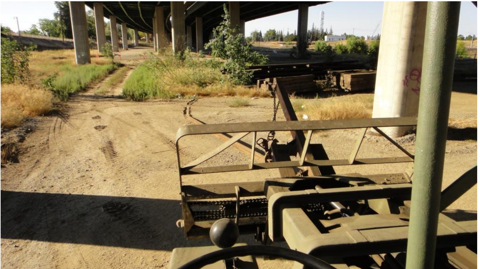
The replacement stick of rail is dragged out from the rail pile
