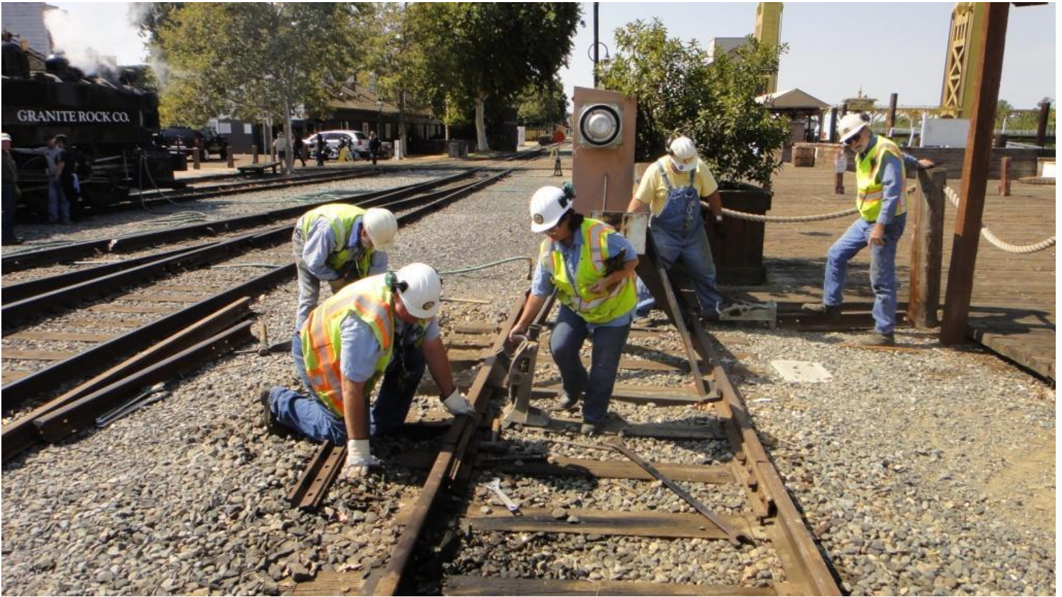
Using a track-jack and a piece of broken rail, Mike F. and Alan shove the south end of the Business Car Track back into alignment. Pam gets another track-jack to lift the rail slightly in order to get all the bolt holes to line up
