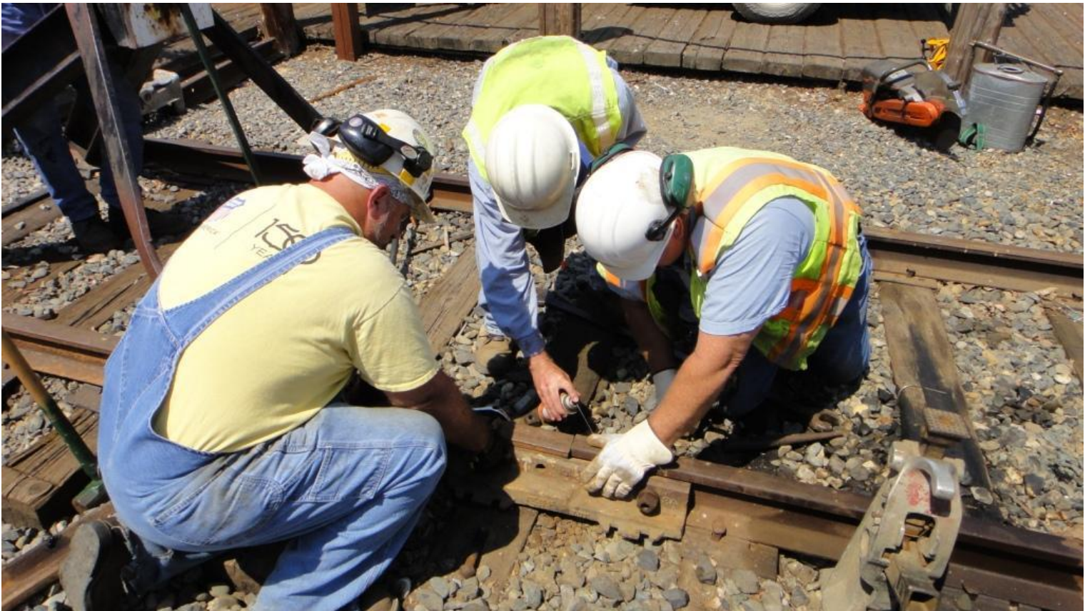
Mike F., Mike M., and Chris "Kroil" the bolts at the joint
