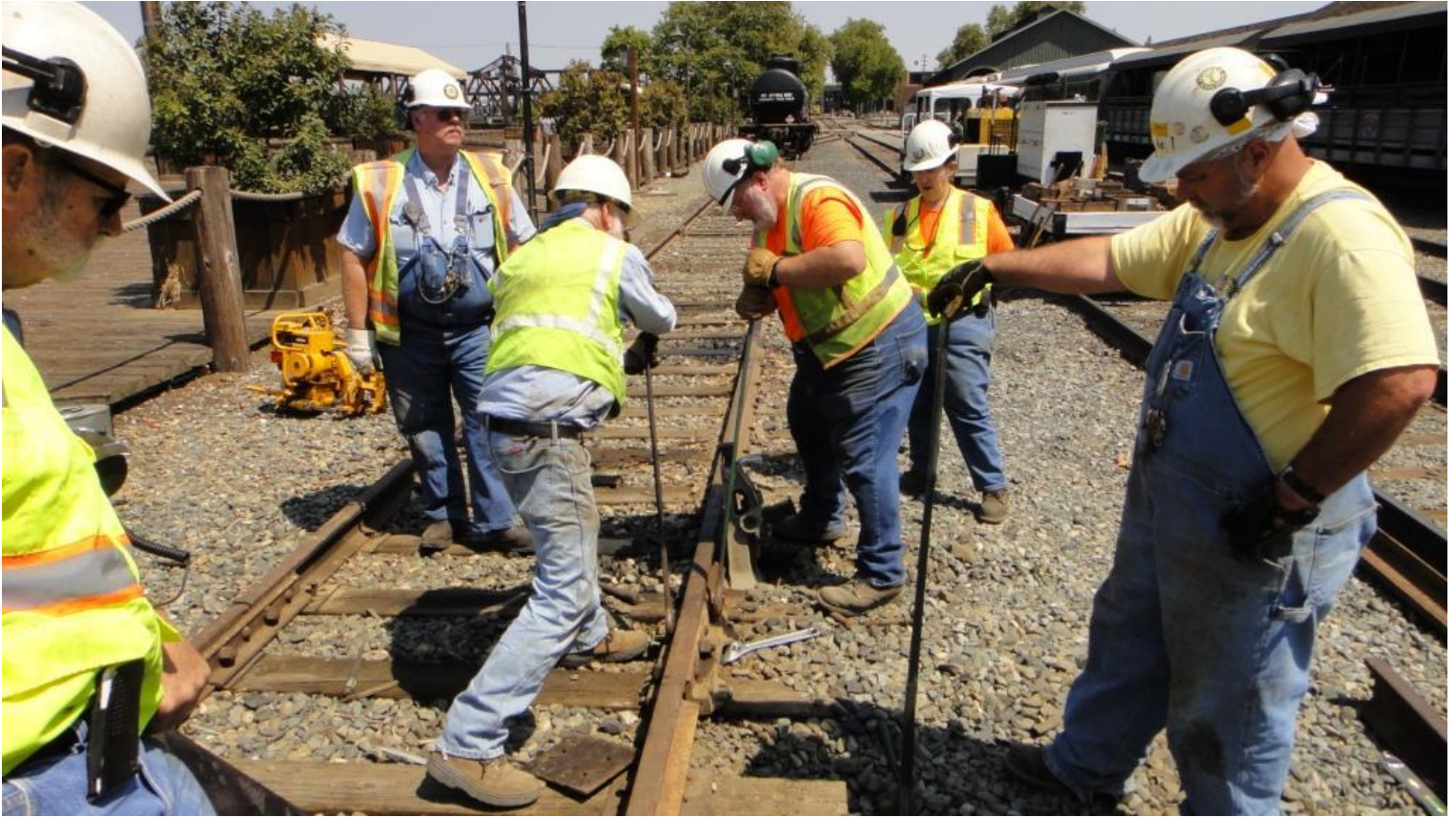
The final step: Mike M. and Frank tighten the bolts
