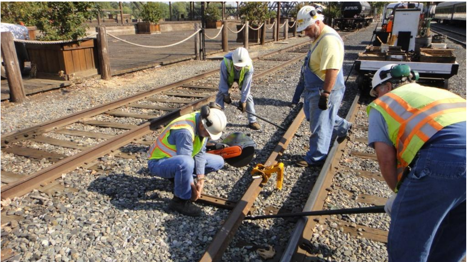
Chris and Mike M. lever-up the new rail while Alan puts a joint-bar under it to make room for the rail-saw blade to cut through the base
