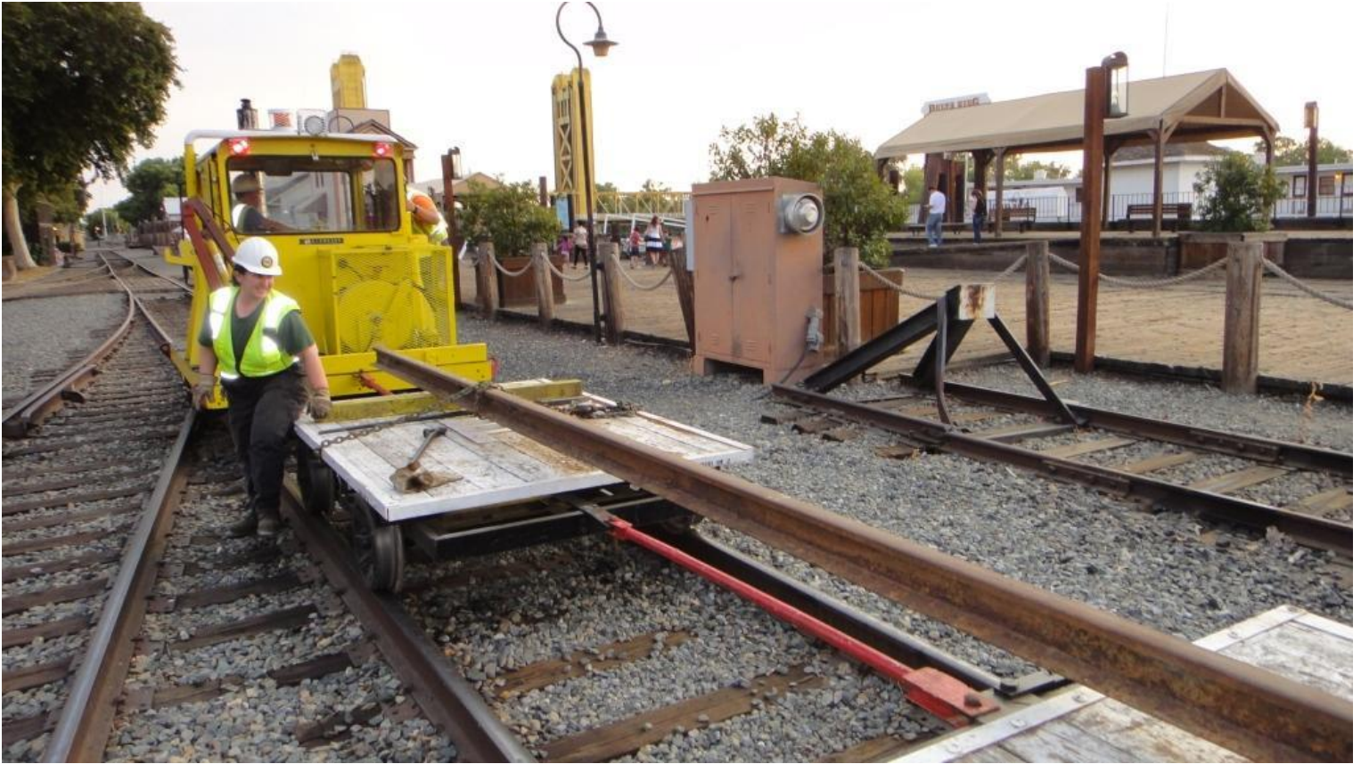
The new rail arrives on site
