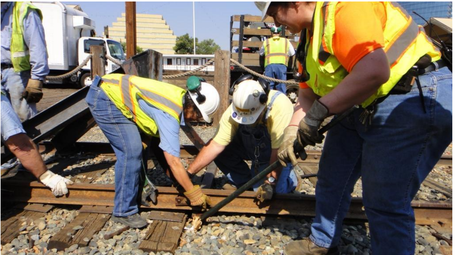
Heather levers-up the rail as Pam and Mike F. line the bumper bracket to bolt it in place
