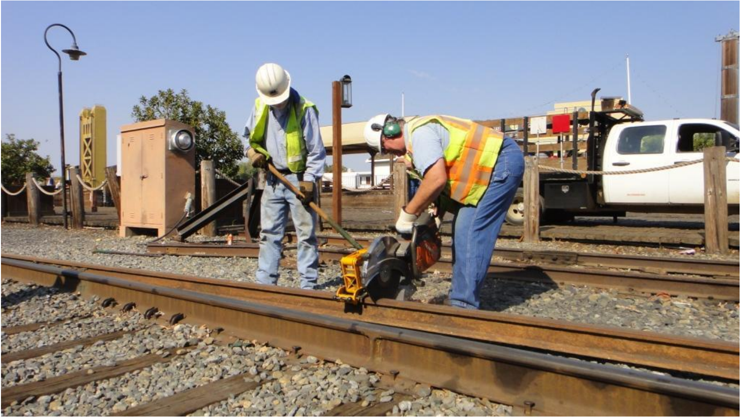
Mike M. places a shovel behind the rail-saw as a shield for the sparks as Chris cuts the new rail to size
