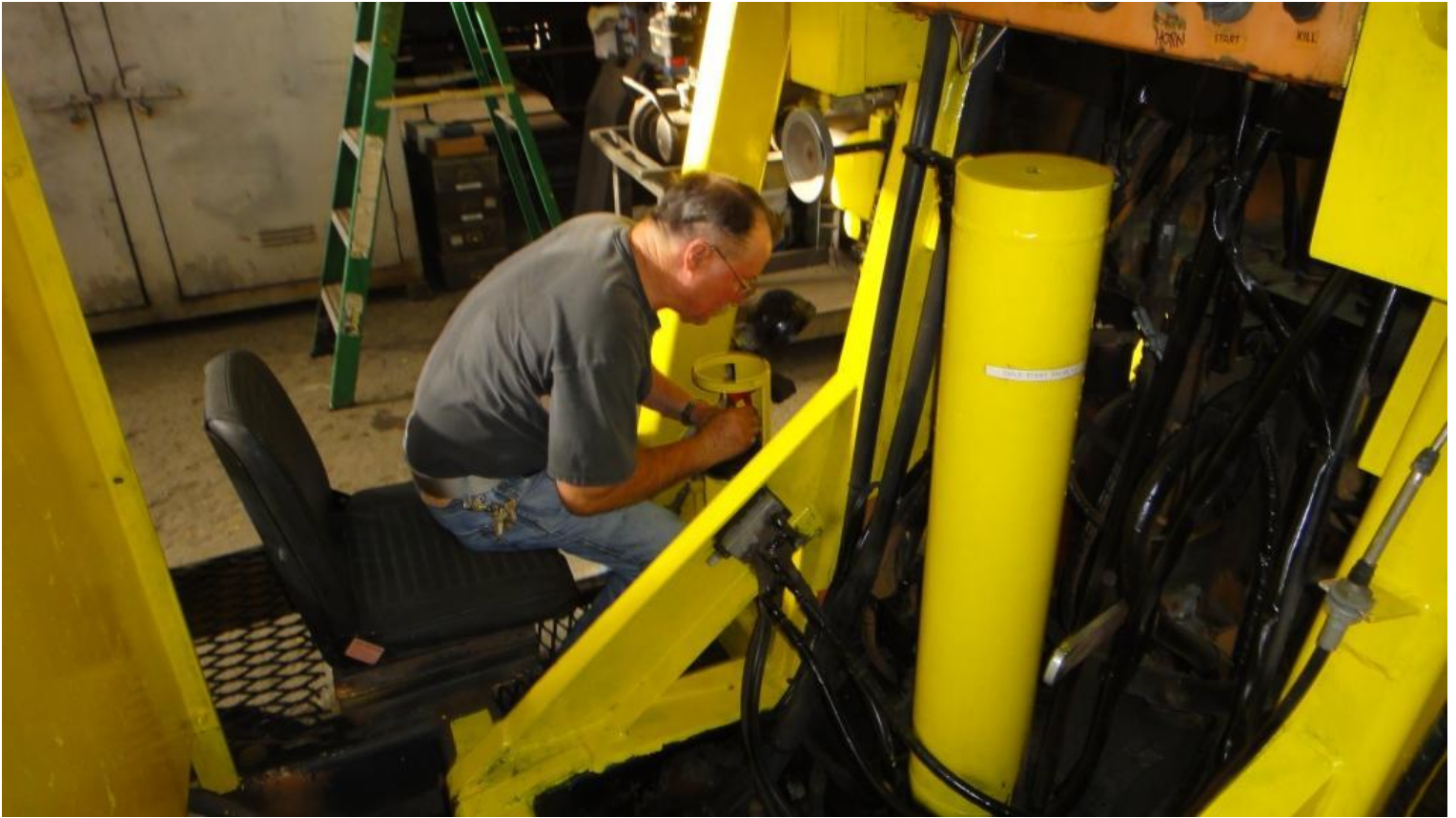
Mike H. installs the multi-directional joystick control valve for the Super "B" Spiker
